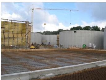
Construction of a biogas plant. Picture: Ch. Boese
